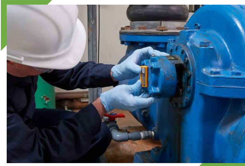
Figure 17. Application of Fluke 3561 FC vibration sensor in industrial pumping systems
