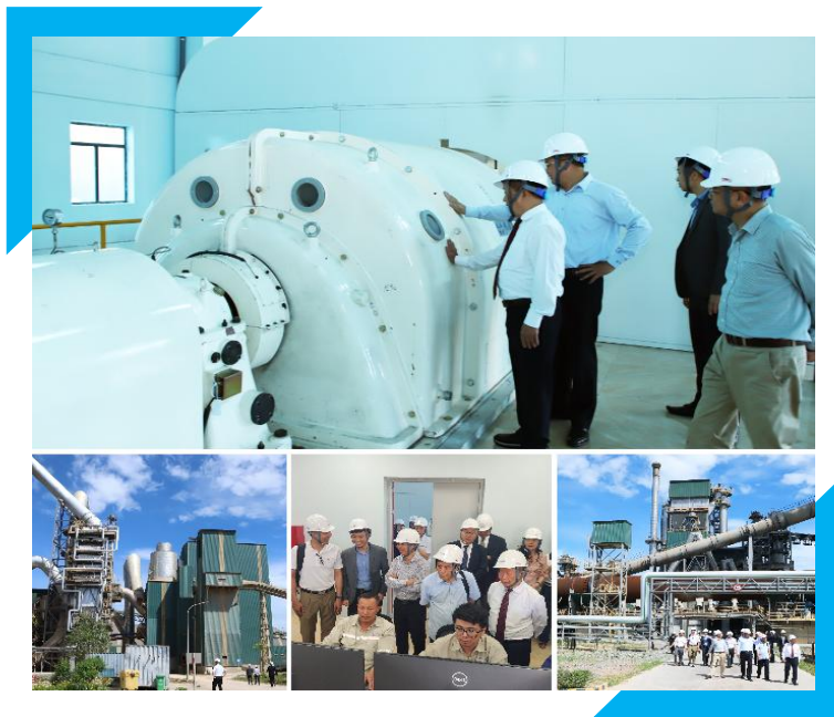
Figure 1. Waste heat recovery system from the emission process at Tan Thang cement factory
