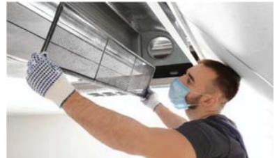
Dirty coils or filters increasing pressure drop in the system.
